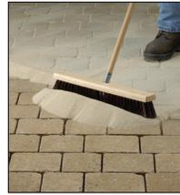
2. Using the street broom, fill joints completely. Sweep sand over short distances.
