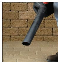
10. On textured pavers, use the blower to blow the excess water off the surface and into the joints.
