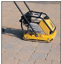
5. Pass the plate compactor over the entire surface a second time\*.
