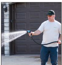
9. Starting from bottom of the slope, quickly shower a 20 m<sup>2</sup> (200 sq. ft.) section to set the sand. Immediately afterwards, wet the same section for **30 seconds**.
